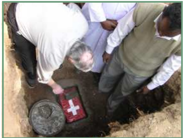
Fr. Greg (with trowel) laying foundation stone.
