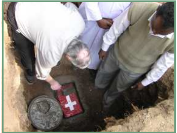
Fr. Greg (with trowel) laying foundation stone.
