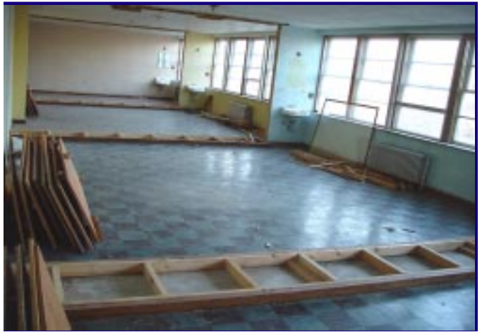
Wood paneling being saved from third floor dorms and library.
